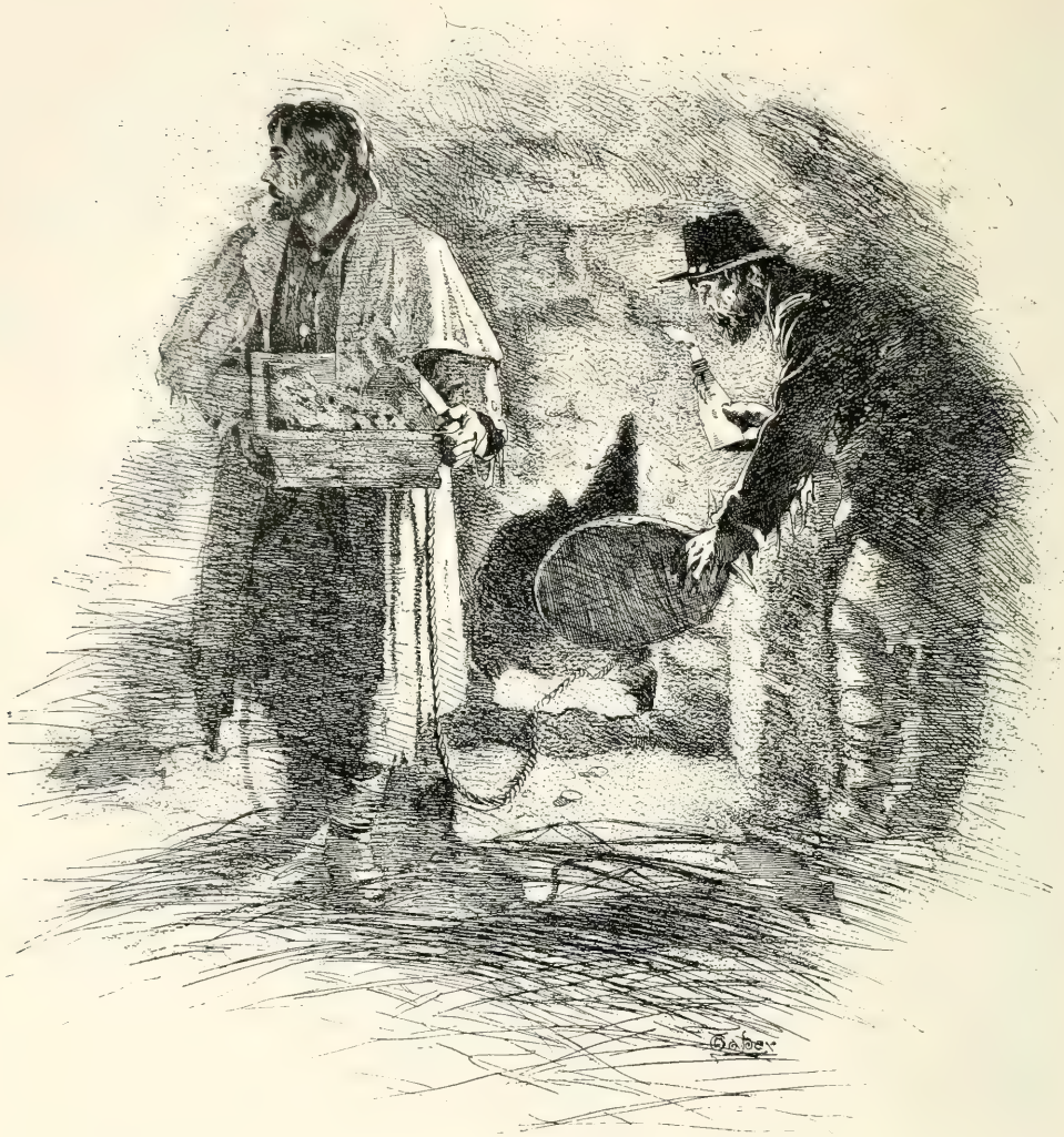
WORKING AT THE TUNNEL.
